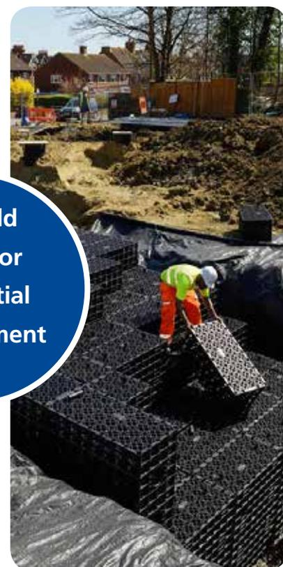
Working closely with Pentland Homes, Polypipe provided a 2700mm Ridgistorm-XL large diameter piping system and a Polystorm-R geocellular system to attenuate stormwater at the new Folkstone development, Scholars Village.
