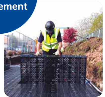
The housing development had previously flooded during heavy rainfall due to interaction between surface water sewers and the water level in the nearby Ouseburn River. To help prevent future flooding, Polypipe's Permavoid system was installed under a recreational area between a road and the river.
