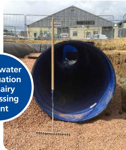
**Stormwater attenuation for dairy processing plant**
