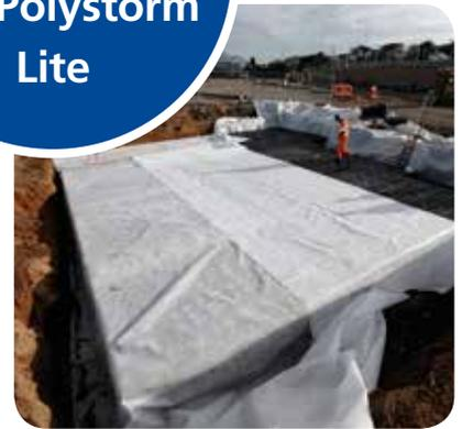
Working closely with the main contractor, Ringway, Polypipe provided a holistic solution utilising its popular Polystorm modular cell system, Ridgidrain surface water drainage pipes and Ridgiduct cable protection products.
