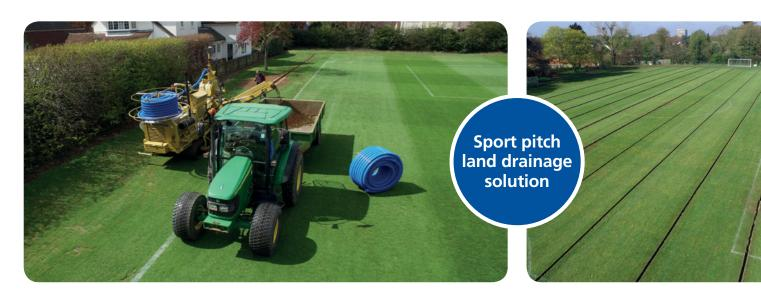
Working closely with main contractor Les Cotton Contractors, Polypipe supplied its PVCu Landcoil land drainage solution in 80mm and 100mm diameters. Installed beneath the pitches at the clubs Playford Road training ground, Polypipe's Landcoil offers significant improvements to the existing pitches which suffered from waterlogging.
