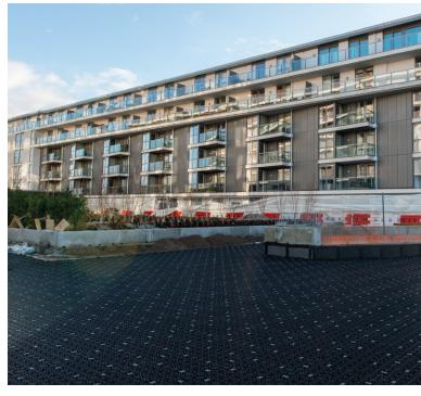
27,600 Permavoid units were used in total, and ideal for the shallow environment available to install the system. And because they are lighter in weight than traditional materials, and have high void ratio, they negated the need for heavy concrete basement tanks. But despite its light-in-weight properties, Permavoid is exceptionally strong – allowing amenity for car parking and maintenance vehicle traffic above, whilst clever water management continues below.
